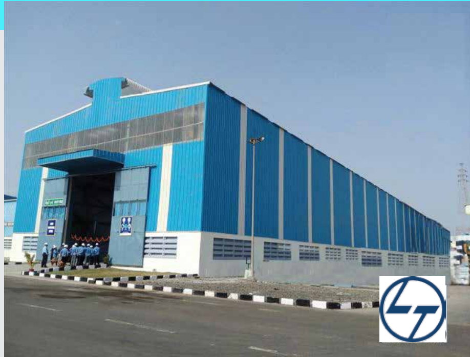
L&T, MHPS BOILERS PVT. LTD, HAZIRA
